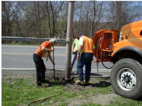
Catch Basin Cleaning
