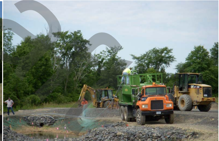
Hydroseeding Stormwater Pond Embankment
