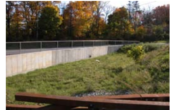
stormwater detention on Golden Hill
