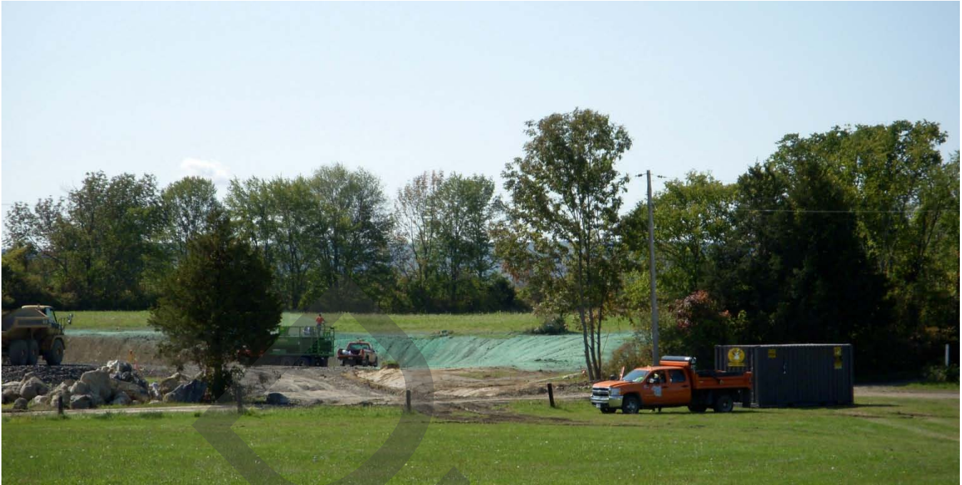
Hydroseeded Slope Stabilization
