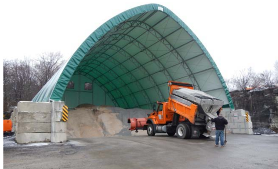
Salt Storage Shed
