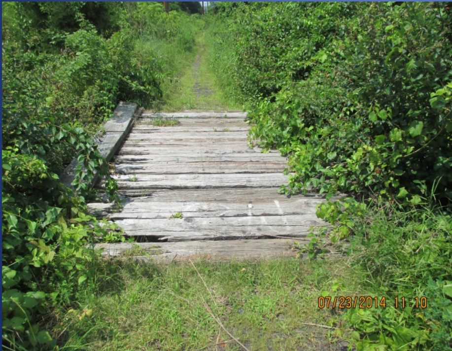
Existing Steel and Timber Structure
