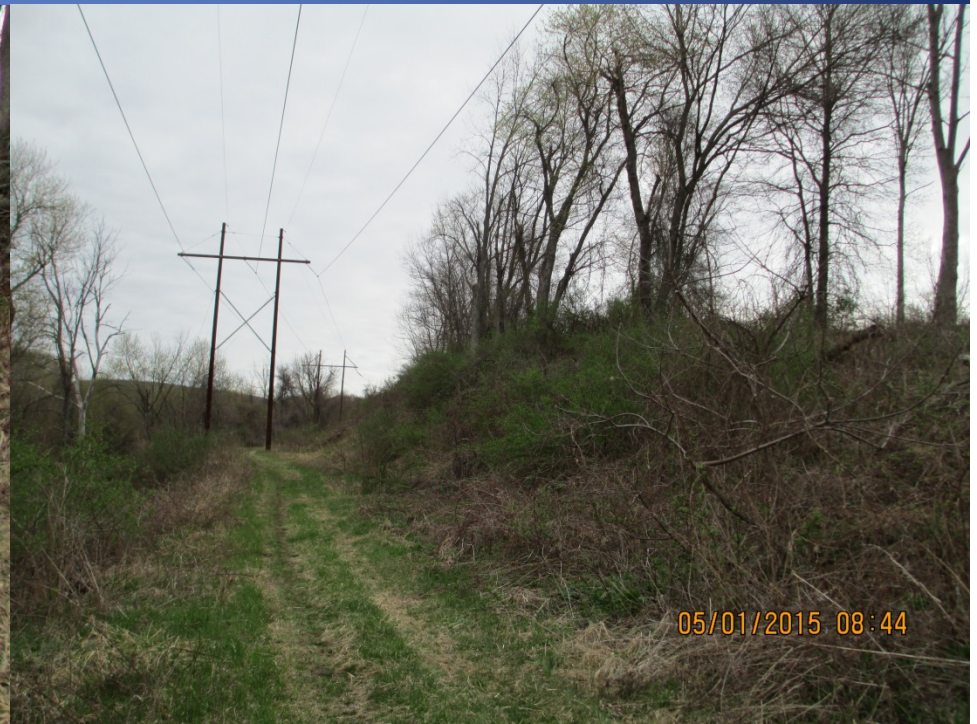
Utility poles owned by CHG&E New Transmission System Planned by CHG&E
