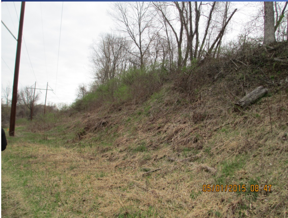
Cut slope along eastern side of corridor
