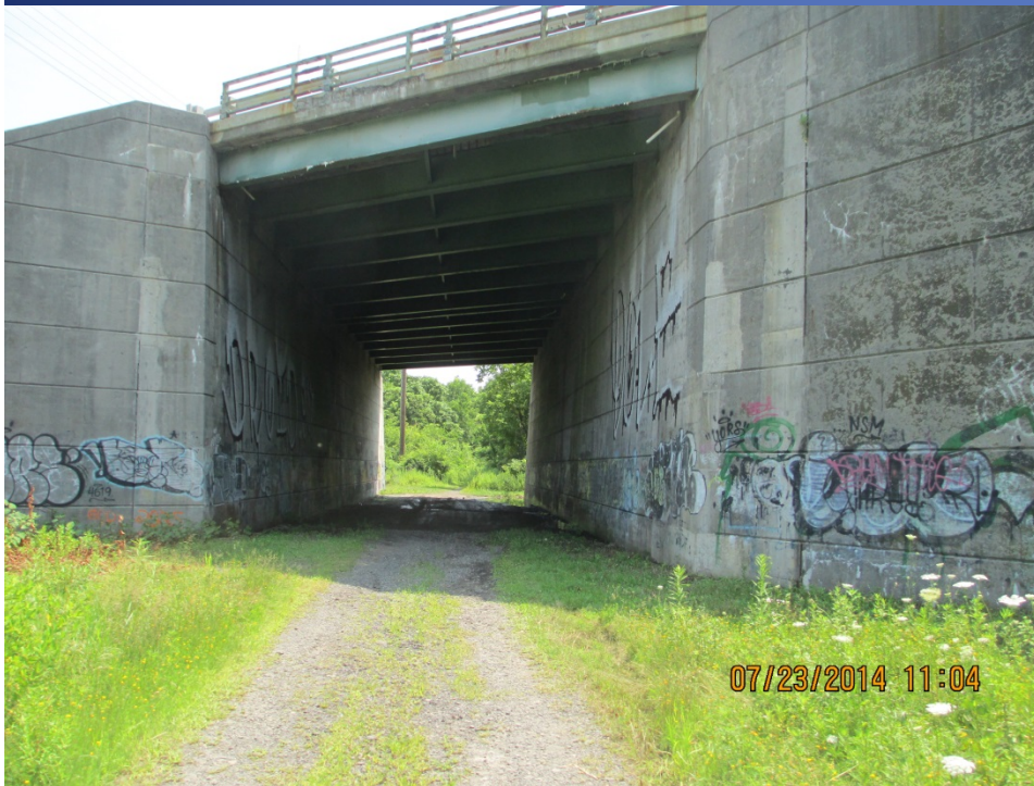
NYS Thruway Underpass – Coordination with NYS Thruway on-going
